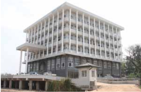
Auditor General Department Constructed under World Bank Assistance
