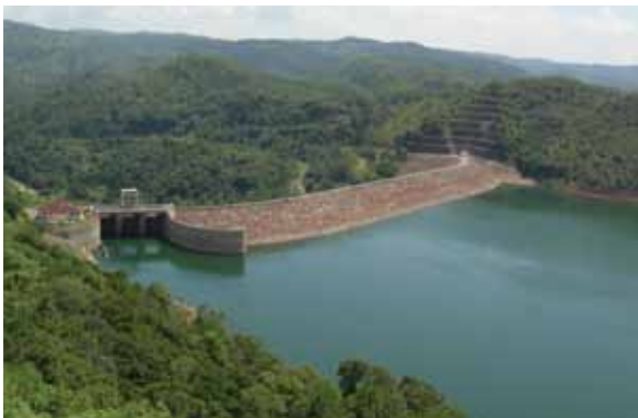
Samanalawewa Hydro-power Project
