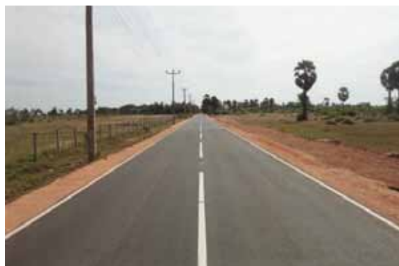
Reconstructed Kalkudah Road under Priority Road Project I
