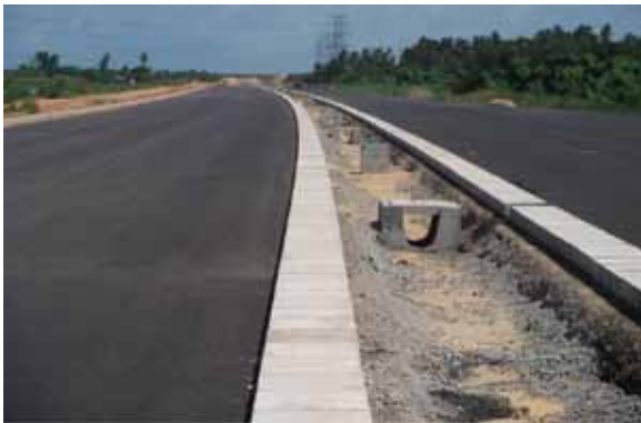
Construction of Colombo – Katunayake Expressway
