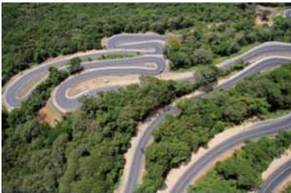
Badulla - Mahiyangana Road rehabilitated with ADB assistance
