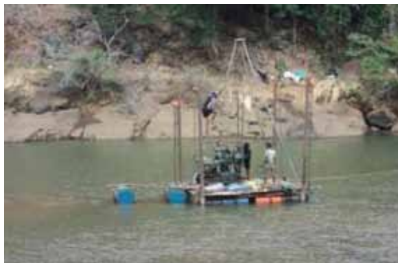
Drilling Testing in Moragahakanda Dam Access
