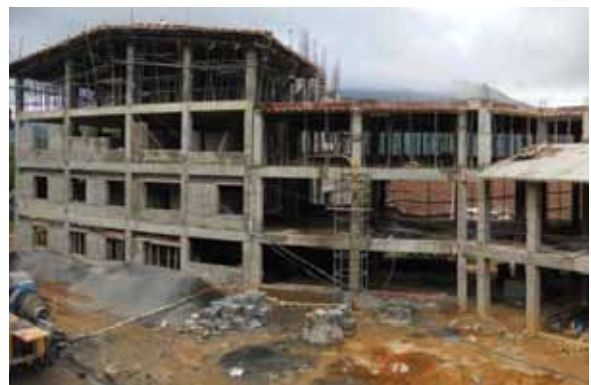
Construction of Dickoya Hospital
