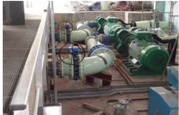
Kantale treatment plant new pumps
