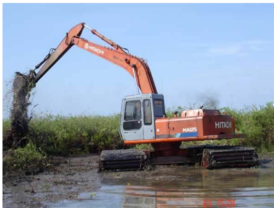
Sea weeds clearing in Raja Ela – Allai Extension Scheme
