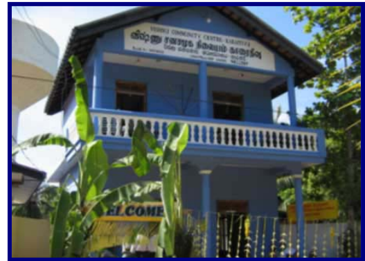
Community Building with Library at Karaitivu – Ampara
