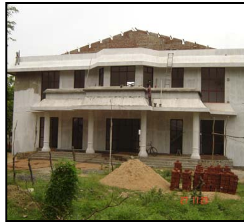
Reconstruction of Hostel - Agriculture Training Centre Vavuniya
