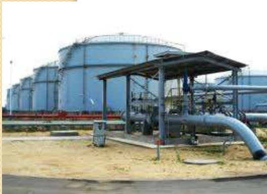
Muthurajawela oil tank project- USD 72 mn The offshore section of the project will have a one-point mooring system and a 5.6 km submarine oil transmission pipeline. The onshore section of the project will have 29 diesel and kerosene storage tanks and all the matching facilities. The Muthurajawela oil tank storage was declared open on 27 May 2004
