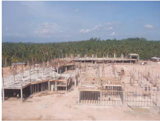
Construction of the Hospital
