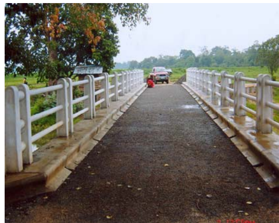
Lahugala Bridge - Ampara
