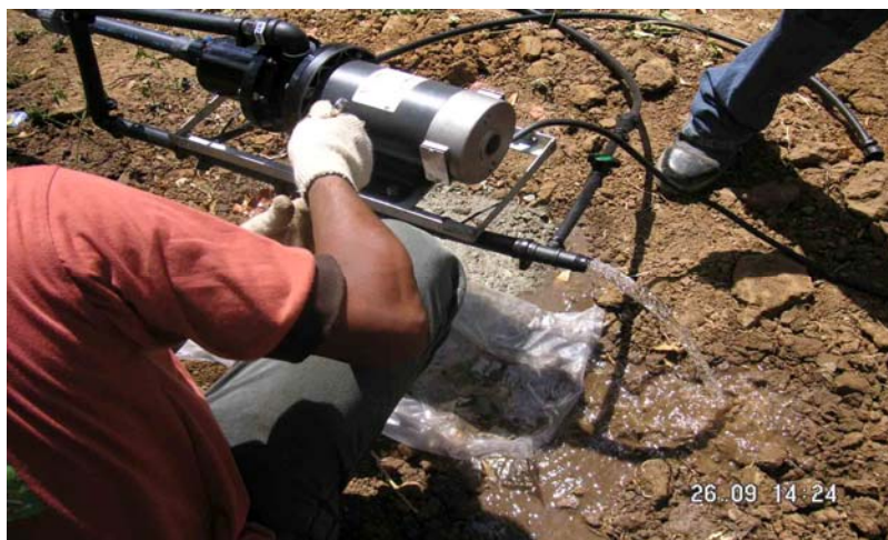
Fixing a solar powered motor for irrigation
