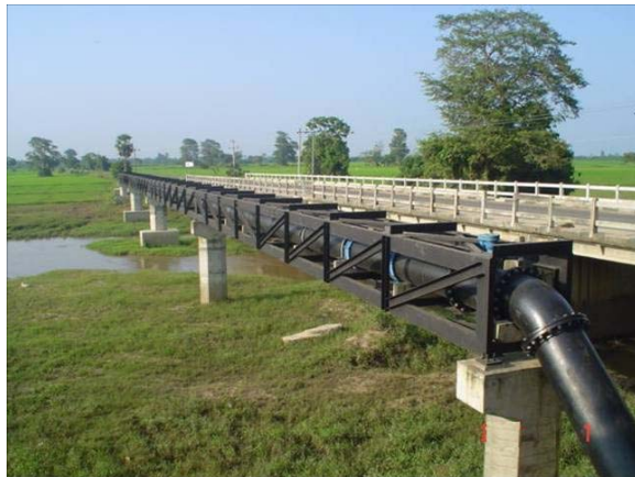
Bridge crossing at Irakkamam
