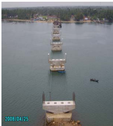
Construction of the Kinniya Bridge
