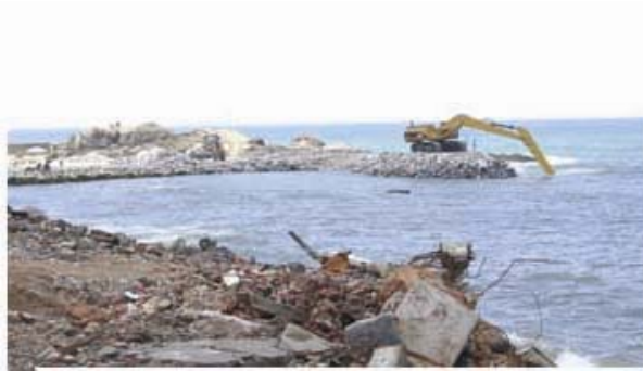
Construction of Breakwater
