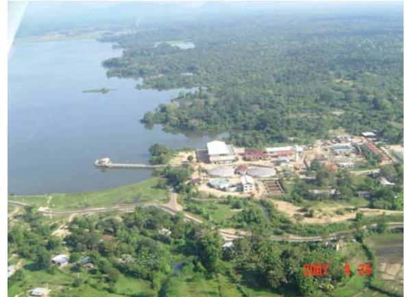
Water Treatment Plant at Ampara
