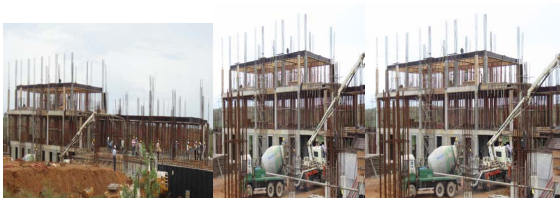
Construction of Administrative Complex
