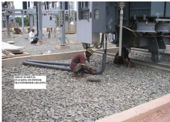
Construction of Aniya Kanda Grid Substation
