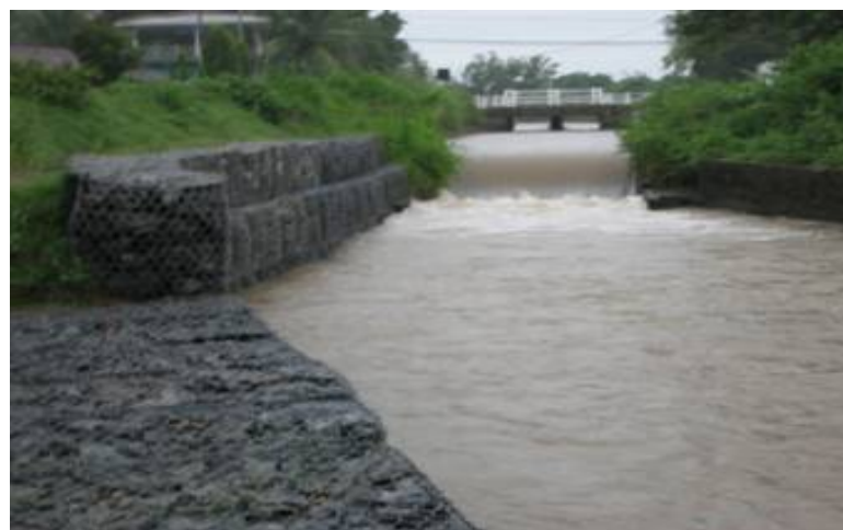
Gabion protection wall - Right Bank - Main Canal
