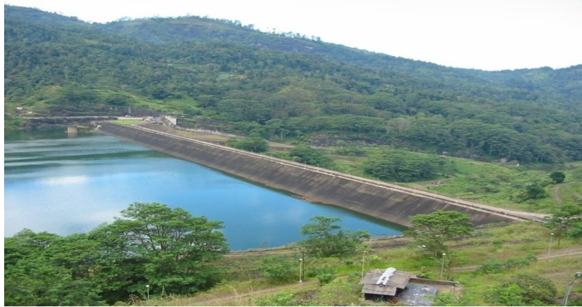
Kotmale reservoir to be rehabilitated under Dam Safety Project
