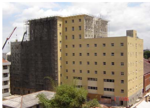
Construction of Neuro Surgical Unit
