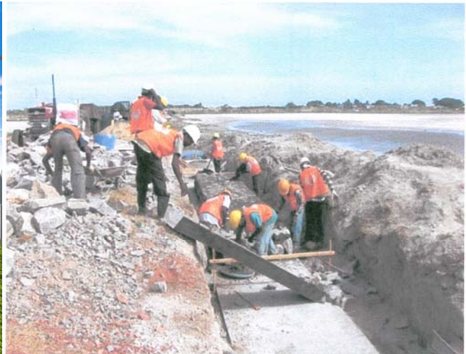
Retaining Wall Construction
