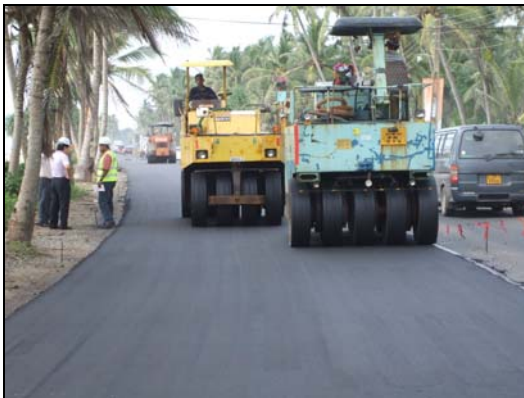
Wearing course laying Ambalangoda- Unawatuna Road
