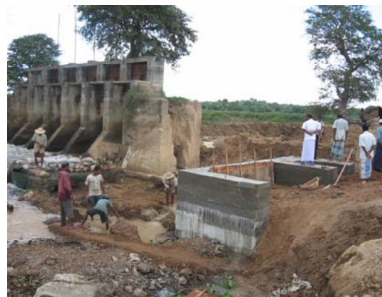
Reconstruction of Vettukadu Irrigation Scheme
