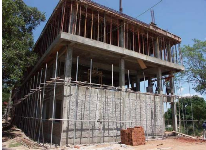
Lecture Hall Building – 3rd Floor Slab Concreted Advanced Technical Institute Ampara
