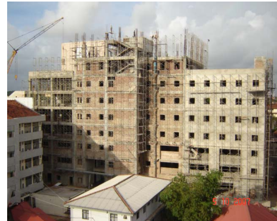
Construction Site of the proposed Neurotrauma building complex
