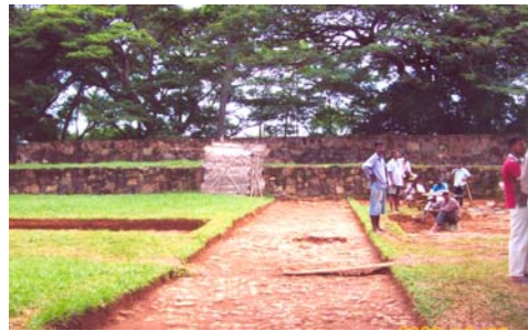
Katuwan Dutch Fort under conservation
