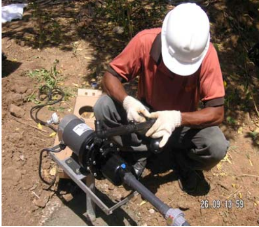
Installation of Solar Drip Irrigation Unit
