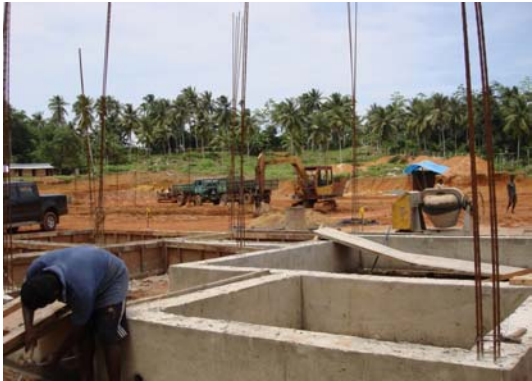
Construction works of Ambalangoda Grid Substation
