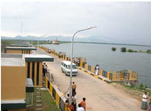
Rehabilitated Spillway at Uda Walawe Dam
