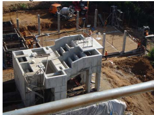
Treatment Plant at Meewatura
