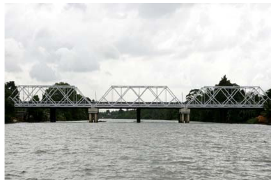
Kelaniya new Railway Bridge
