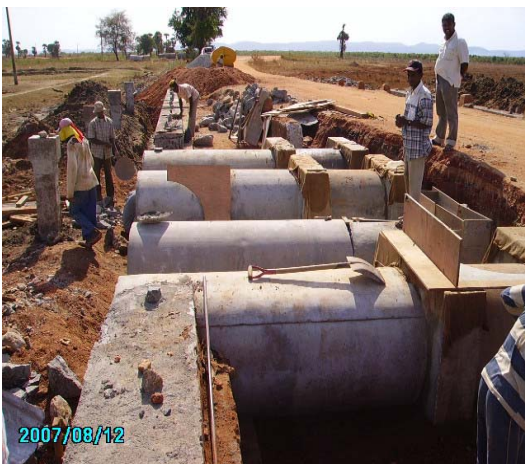
Thampalakamam-Kinniyai Road- Under construction
