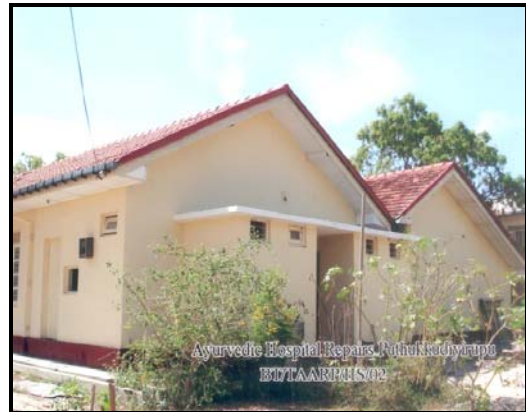
Reconstructed Ayurvedic Hospital – Batticaloa
