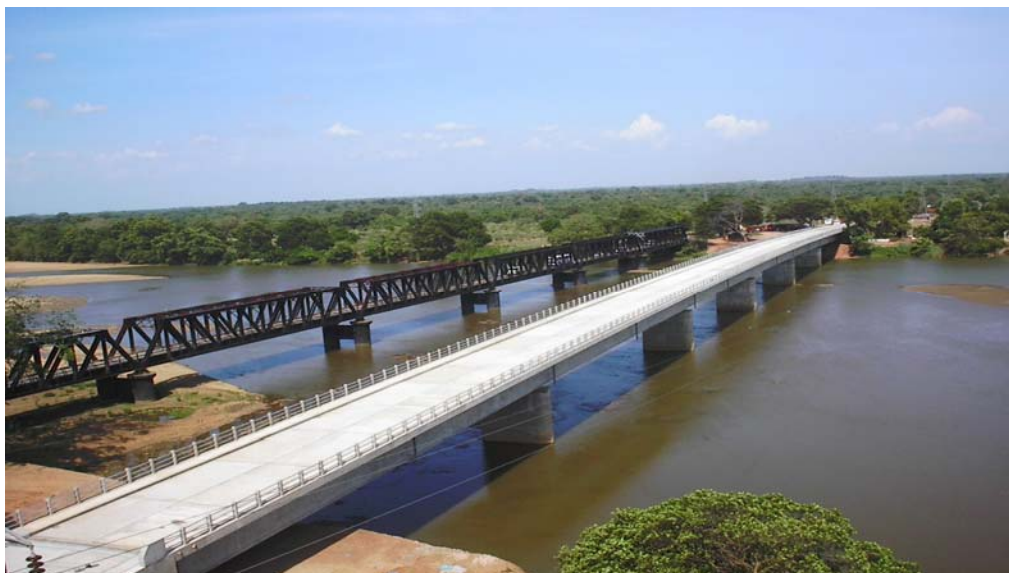
Newly Constructed Manampitiya Bridge
