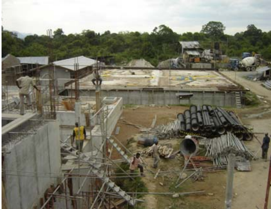
Ampara Treatment Plant
