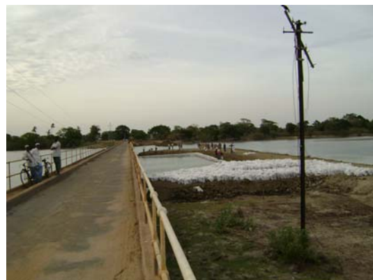
Construction of new bridge
