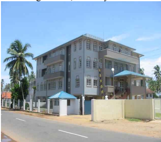
Rathgama Police Station
