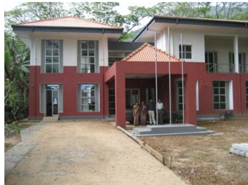
Network Access Center (NAC) - Monaragala
