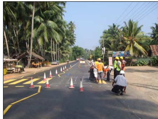
Road marking Katukurunda – Ambalangoda Road
