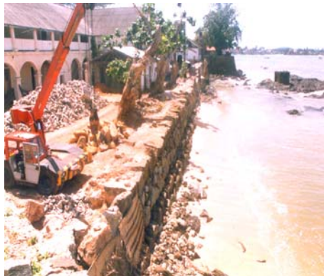
Rampart- Galle under Conservation
