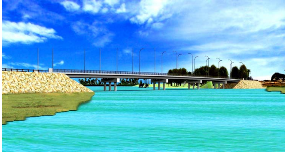
View of the New Arugam Bay Bridge after completion
